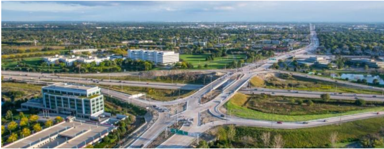
Diverging Diamond interchange at Illinois Route 59 and I-88
