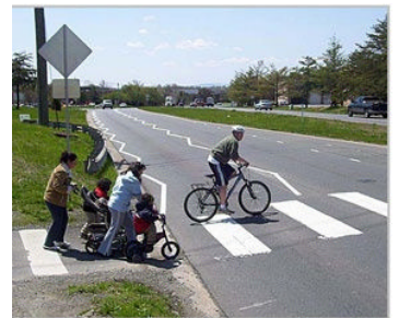
Zig-zag lane edge lines on Sterling Boulevard in Loudoun County, Virginia
