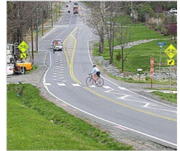
Center of lane zig-zag markings on Belmont Ridge Road in Loudoun County, Virginia
