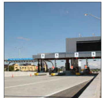
Open Road Tolling (ORT) and cash lanes at the Meyers Road Toll Plaza on the Illinois Tollway's Reagan Memorial Tollway (I-88)
