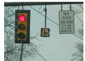
A traffic signal in Ohio includes a separate signal head (to left of NO TURN sign) to confirm to drivers that the presence of the vehicle (in this case for a low volume side street) has been detected.
